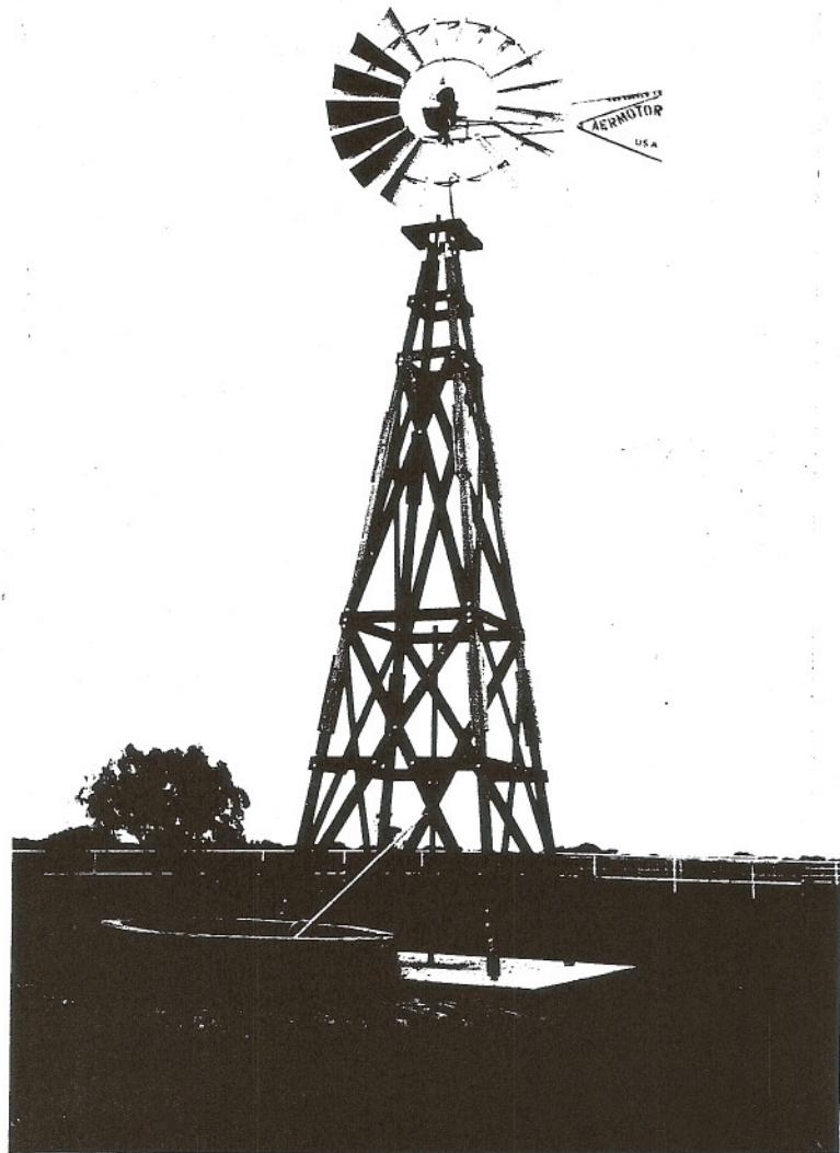
**14 FOOT WOODEN TOWER FOR A WINDMILL WITH A 6 FOOT MILL**
